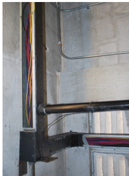
One example of wire management from Fire Service panel to controller.
